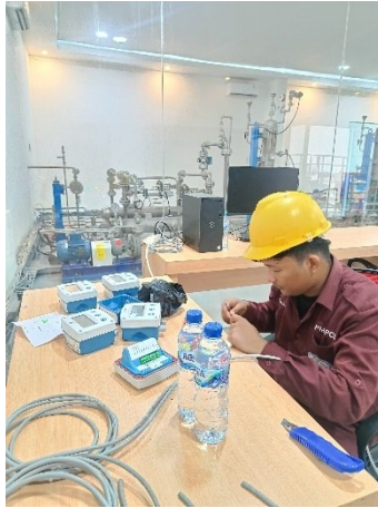
Foto sedang wiring sensor flow rate di PT. Fluid Science Dynamics
