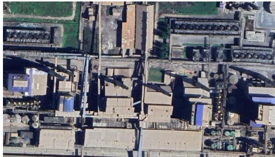
Gambar 2. 5 Peta Lokasi Unit Power Generator 2 (PG-2)
