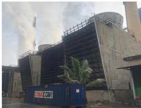
Gambar 3. 16 Cooling Tower
