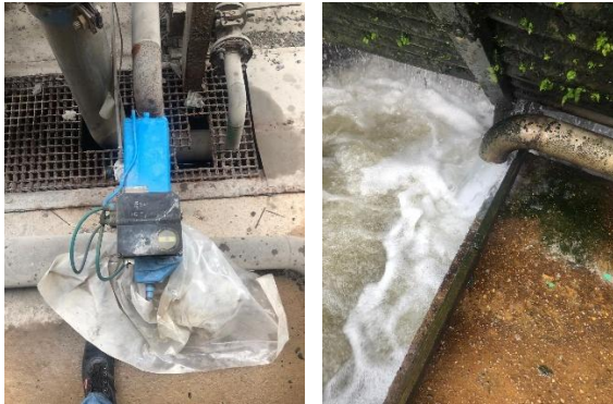
Gambar 3. 29 Control Valve Make-up Water
