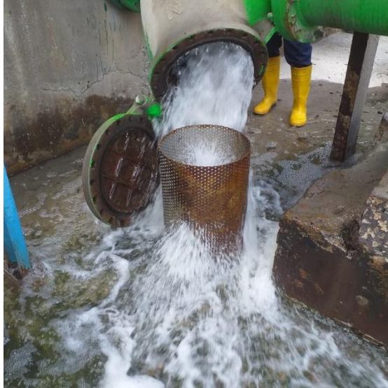
Pembersihan Strainer Cooling Tower
