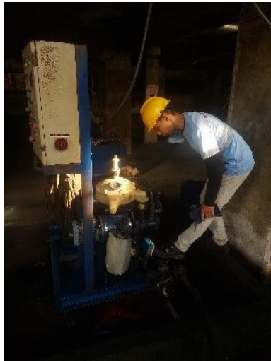
Gambar 4. 13 Start or Stop Oil Separator
