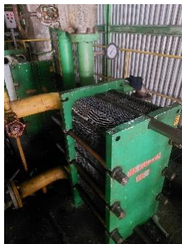
Gambar 3. 13 Oil Cooler dan Oil Filter
