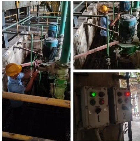
Gambar 4. 14 Change Pompa Condesat
