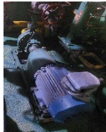
Gambar 3. 11 AC Auxiliary Oil Pump
