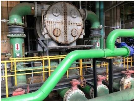
Gambar 4. 3 Condensor Turbin
