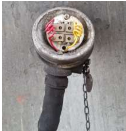
Gambar 4.2 Pengecekan Sensor Thermocouple
