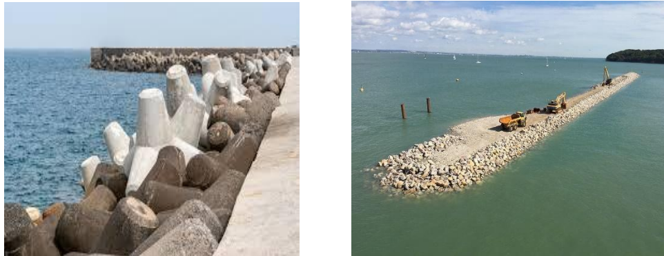
(a) Shore-connected Breakwater, (b) Offshore Breakwater
