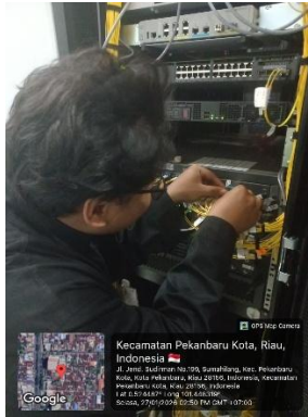
Gambar 4. 3 Pergantian Modul SFP
